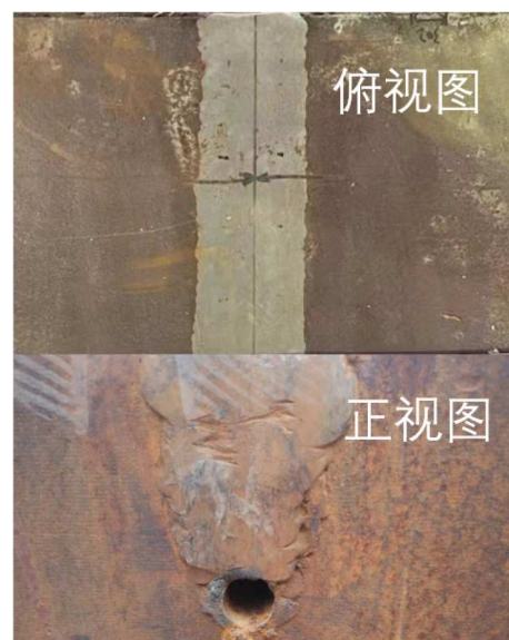
图1 焊接区 Figure 1 Weld zone.
