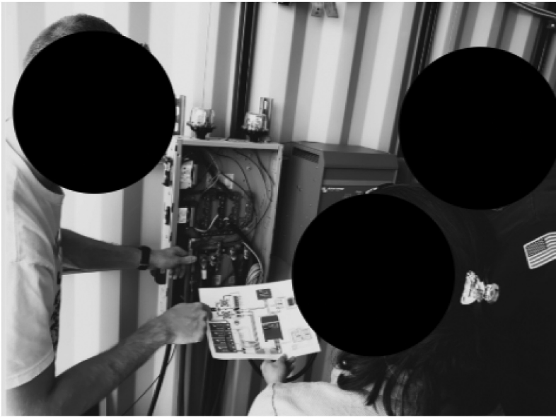
Figure 3. Hands-on practice in commissioning off-grid microgrid.
